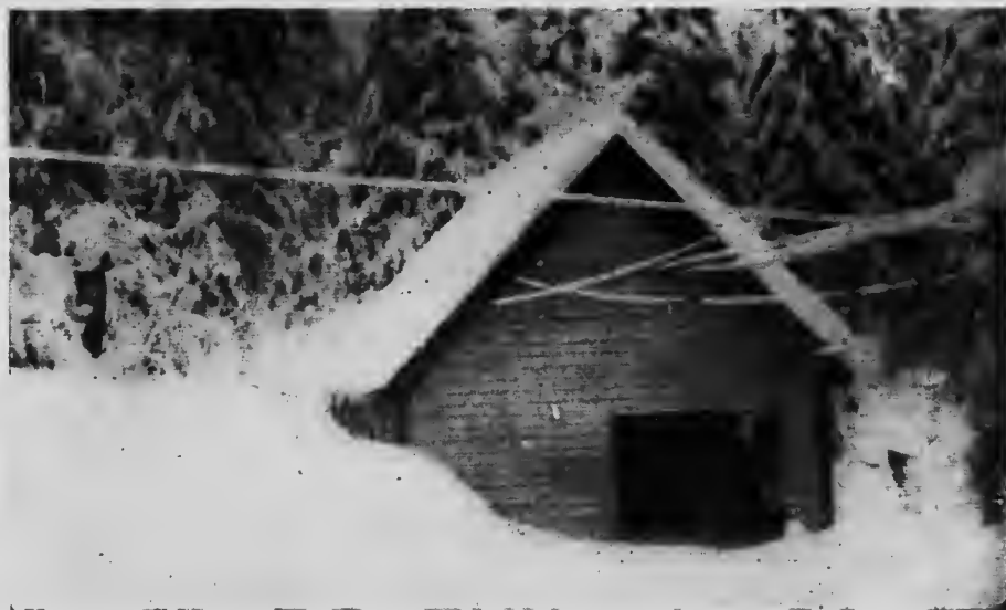
Illicilliwaet River Development at Glacier. View of Power House in Winter.
